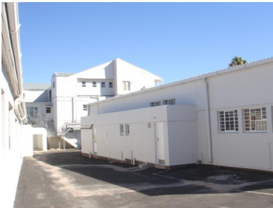
VIEW FROM THE SECURE PARKING AREA AND STAIRS TO TOP FLOOR.
