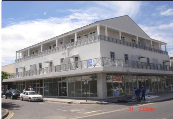
VIEW OF 2 OFFICE FLOORS LIBRI LANE AND VICTORIA STREET
